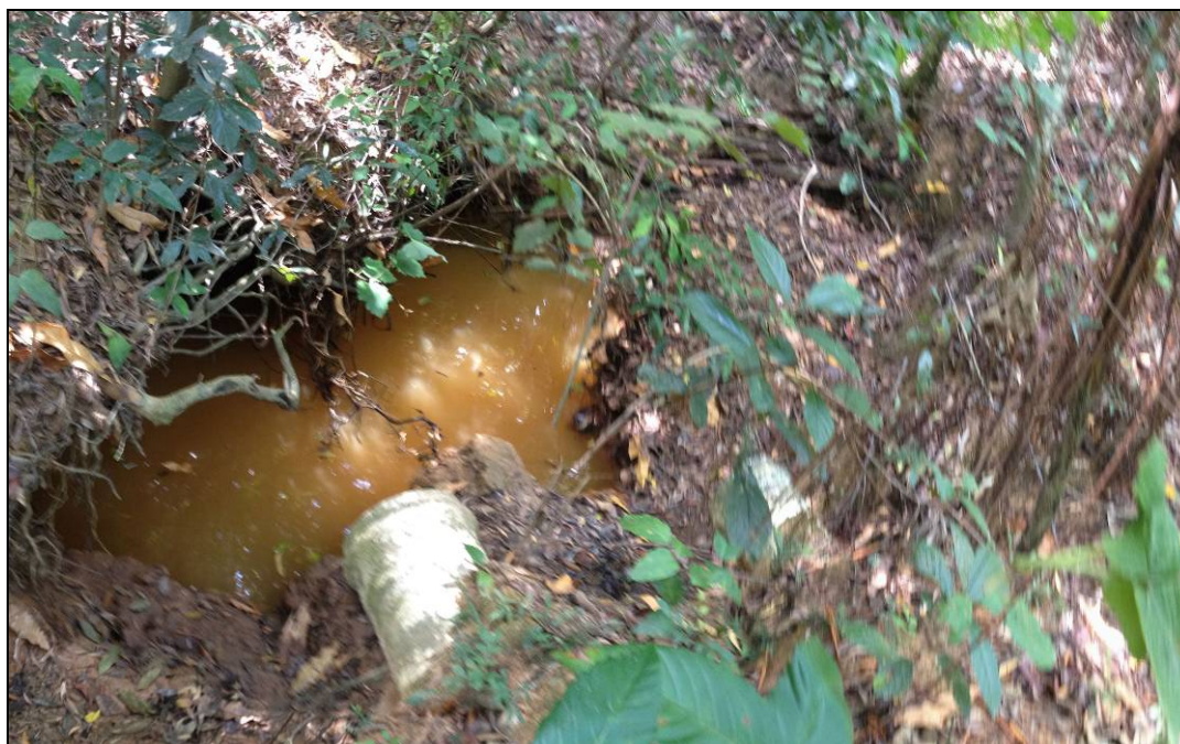
Figure 9: Scour hole on downstream side of culvert
