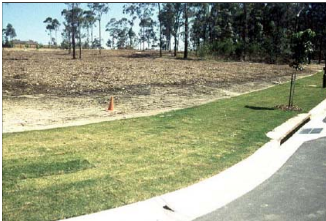
Figure 12: Use of a grassed filter strip for erosion control and sedimentation
