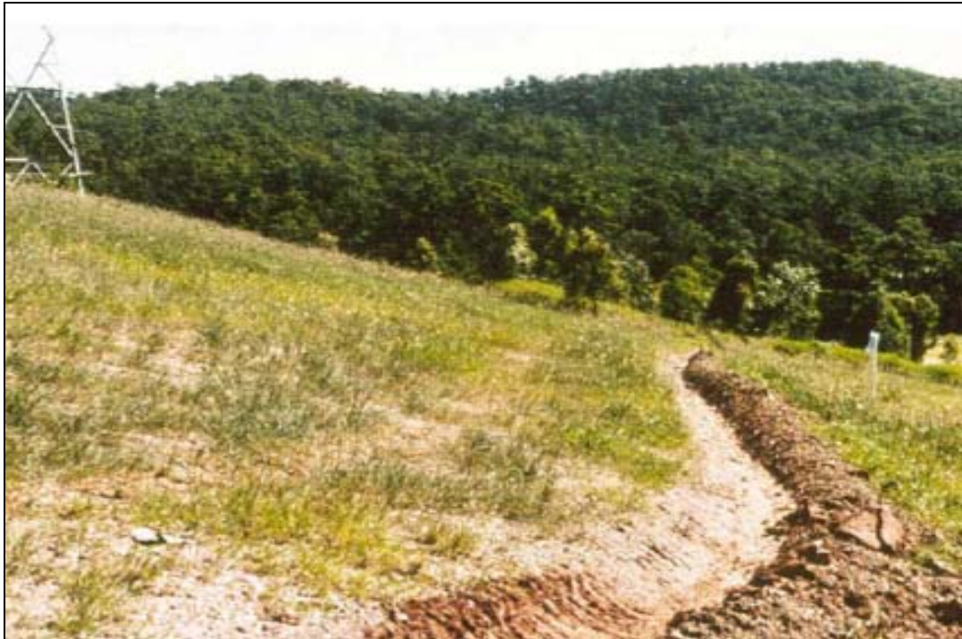
Figure 10: Unlined catch drains to reduce erosion processes
